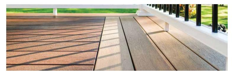
Color-matched plugs camouflage screw heads across the deck surface, stairs and perimeter boards.
