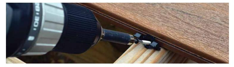
For all other Phantom and Tiger Claw TC-G fasteners, the clip is installed into the groove and a screw is driven into the joist at an angle.
