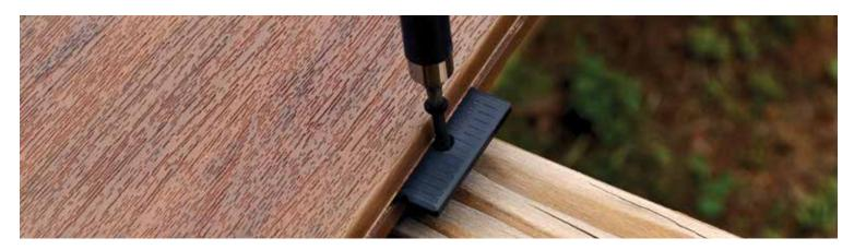
For the Phantom Universal fastener, the clip is installed into the groove. Then, a screw is driven straight down into the joist (90° angle).
